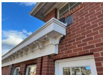
back edge of flat roof see pulling from edge
